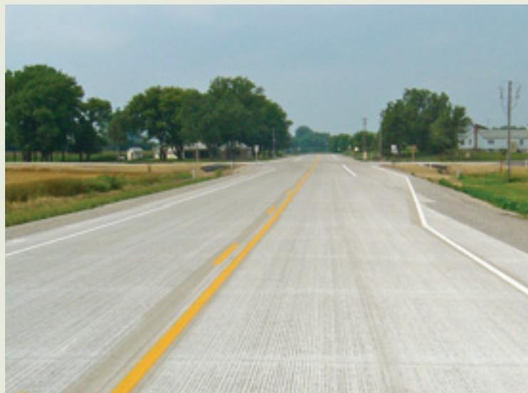
Top to bottom: Michels used about 15,500 cubic yards of concrete to pave an overlay 7-1/2 inches deep and 30 feet wide over 4.25 miles of highway.
