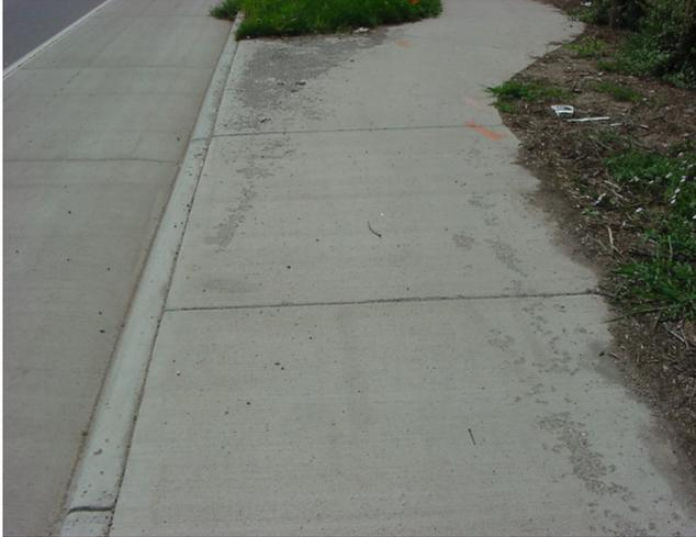
This picture is an illustration of a property owner that struggled with snow removal over the last two winters. Two visible snow lines can be seen on the sidewalk. The area on the left scaled where snow was stored for a long period at the sidewalk transition away from the roadway. And, the area on the right scaled where the snow was left in place due to the large volume that needed to be moved because of the snow plows.
