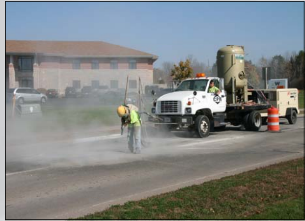
Sandblasting the repair
