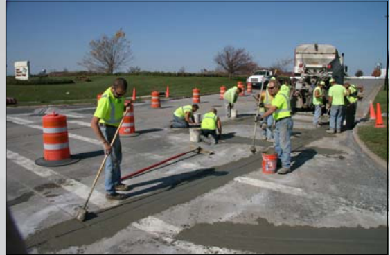
Brooming slurry around edge of repair
