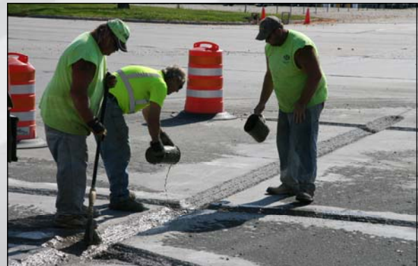
Adding slurry to repair area to promote bond
