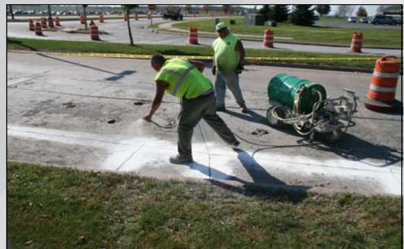
Curing of completed repair
