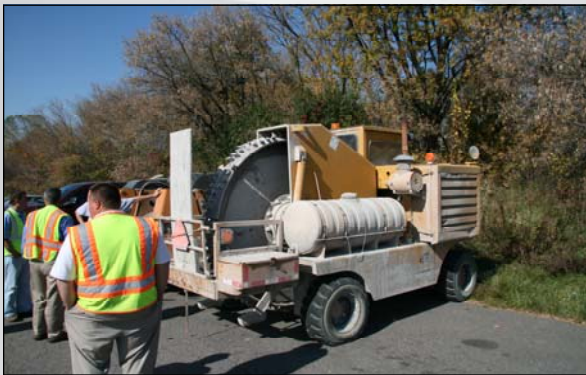
Vermeer used to grind the deteriorated concrete from the repair.
