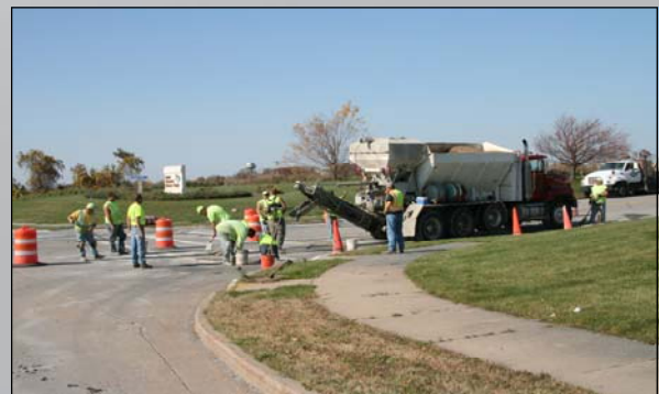
Volumetric mixer used to place concrete in repair
